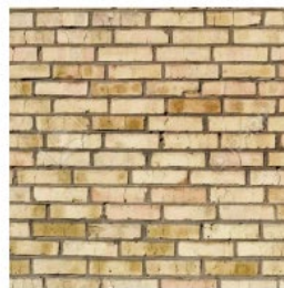
MW-01 Existing brick to be stripped
